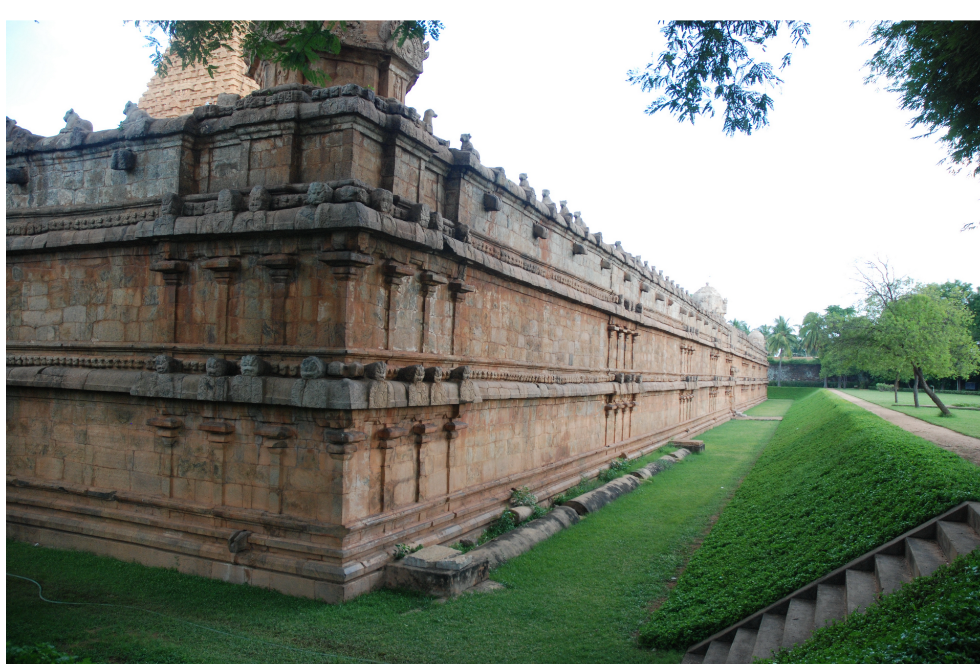
West view from north-west corner of enclosure
