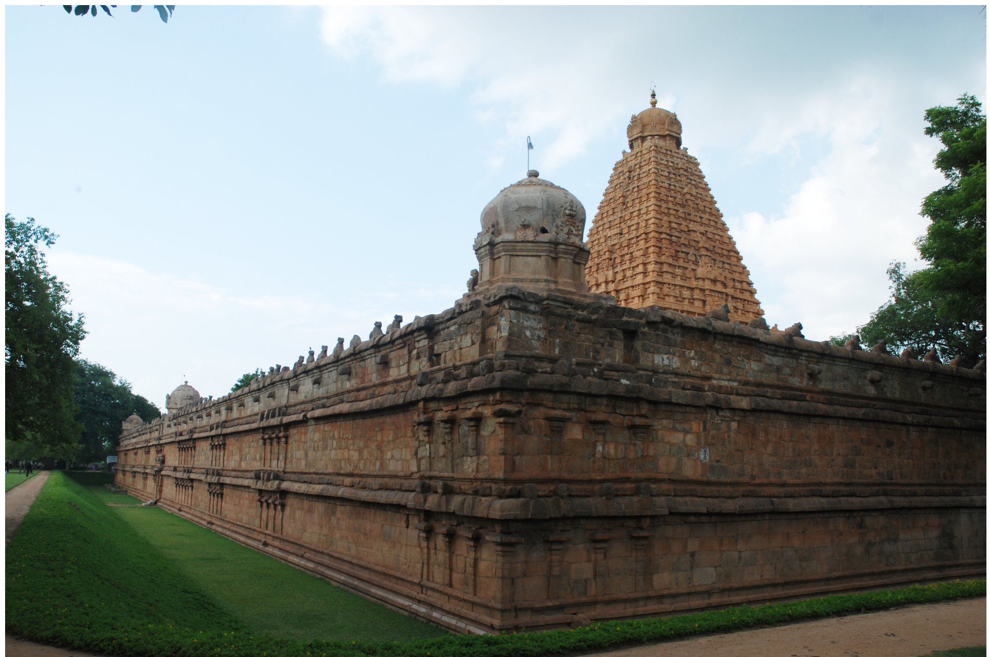
West enclosure view from south
