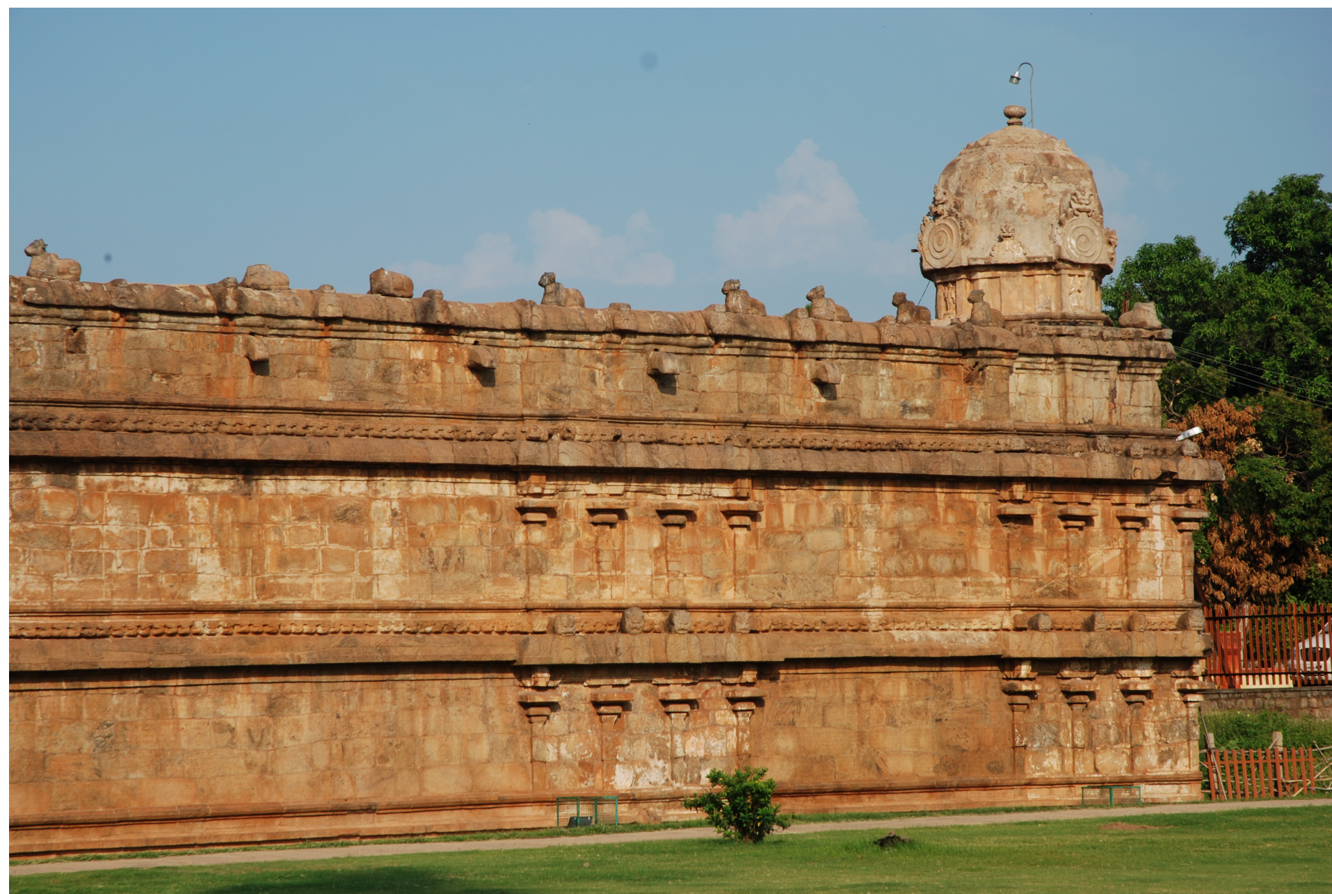
West view from north-west corner of enclosure
